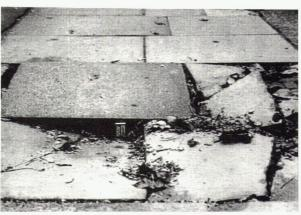
Broken paving stones, frequently caused by parked cars, are a significant source of pedestrian accidents
